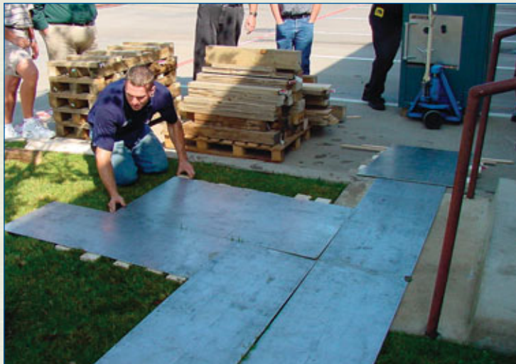
I. Plating over grass with 2 X 4's and aluminum plates.
